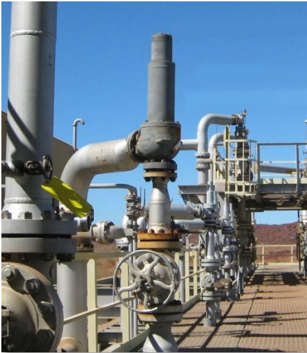
Fig. 1 - Relief valves can produce high AIV
